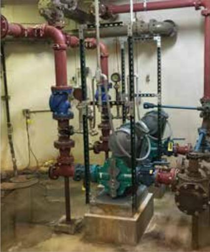
The City of Otsego WWTP installation of NETZSCH TORNADO® T2 Rotary Lobe Pumps.
